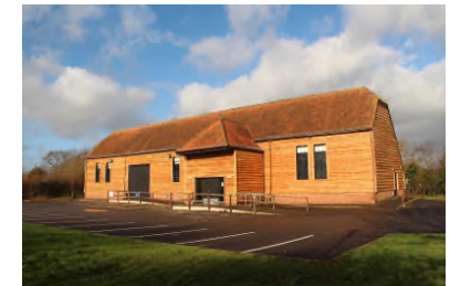
The "re-clad" Barn
